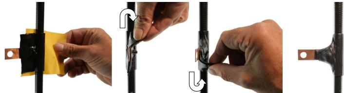
Remove the second covering paper. Fold both overlapping edges in opposite direction of the screw head. Press and form the butyl sealing compound over the complete of-site screw thread to a seamless transition.
